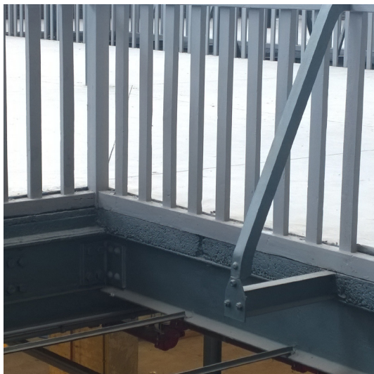
Figure 1: floorbeam [E-F] protruding mould stabilizing railing own picture
