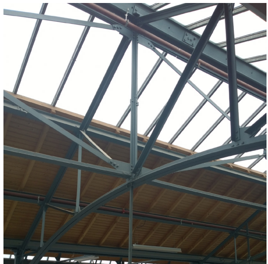
Figure 2: drawbars between central trusses own picture
