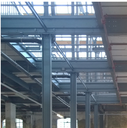
Figure 1: first floor column [E6] directly on primary beam own picture
