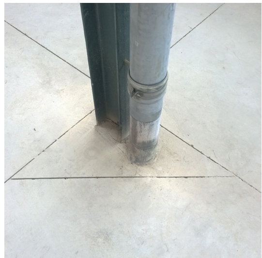
Figure 2: clear seams in first floor [H2] own picture
