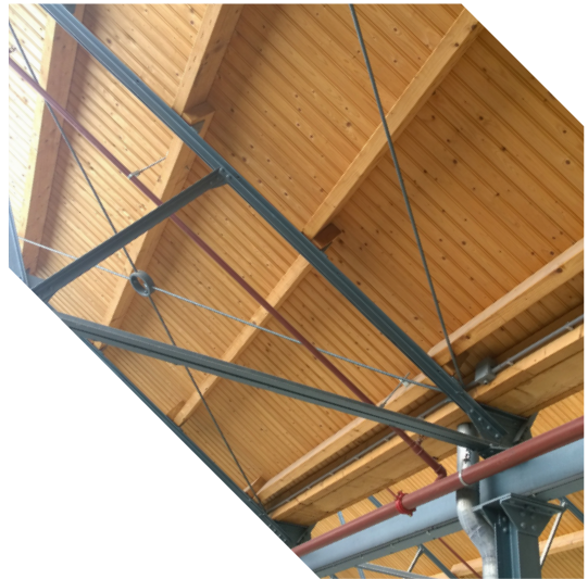
Figure 2: drawbars between trusses own picture
