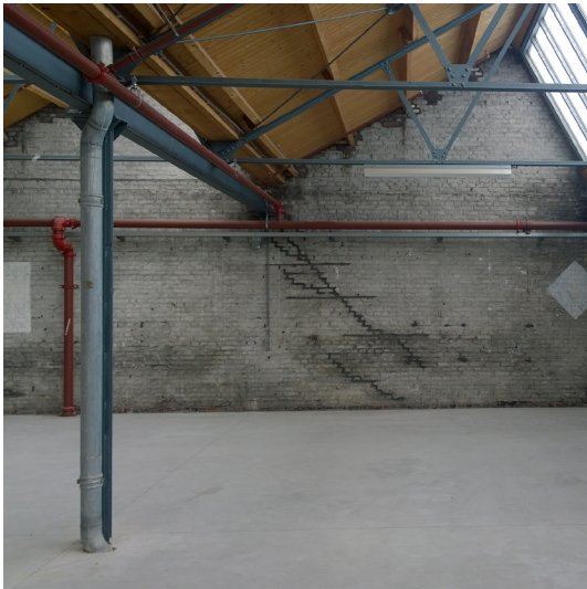
Figure 1: connection of truss to column own picture
