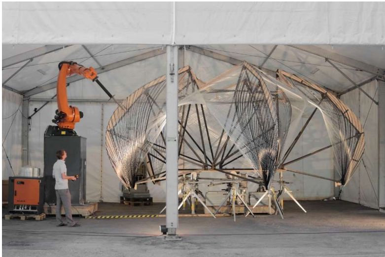
Figure 2: The robotic fabrication process of Research Pavilion 2012
