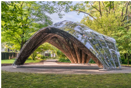
LivMatS Pavilion 2021 2021 ICD Research Buildings / Prototypes Botanic Garden Freiburg, Germany
