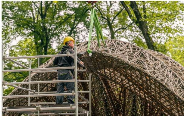
Figure 21: Placement of the fibrous elements livMatS Pavilion / ICD/ITKE University of Stuttgart (2022, 14 Aug). ArchDaily. Accessed 10 Dec 2023. < https://www.archdaily.com/966168/livmats-pavilion-icd-itke-university-of-stuttgart > ISSN 0719-8884
