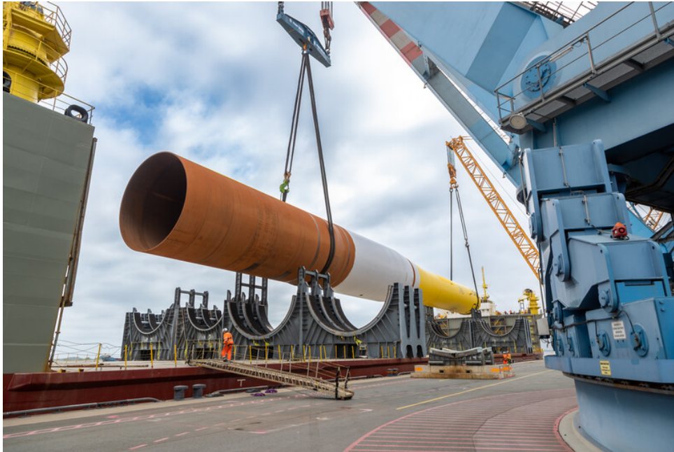
Figure 17: Illustration of the monopile.
