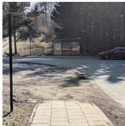
84. Lack of crossing to PT stop.
