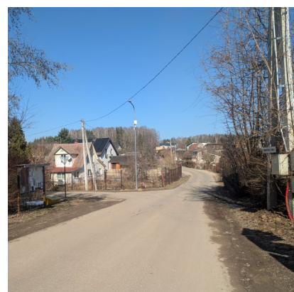
93. Oversized road with no lighting
