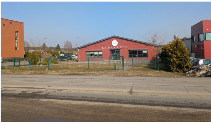
82. Uninviting environment around bakery at local centrality.
