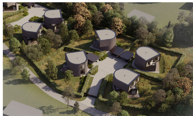
Figure 14. Suburban gated community project near Vilnius.
