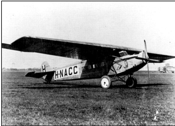
Figure1.3: Fokker F-7; example of a passenger aircraft with a welded framework structure and a plywood/fabric covering developed in 1924. [ www.dutch-aviation.nl ]
