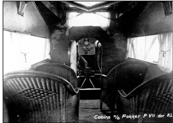
Figure1.3: Fokker F-7; example of a passenger aircraft with a welded framework structure and a plywood/fabric covering developed in 1924. [ www.dutch-aviation.nl ]
