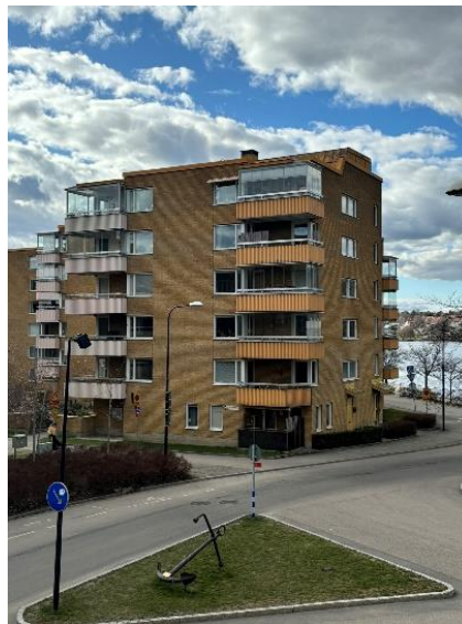
Figure 5: Residential block Gröndalsvägen (own work, 2025)
