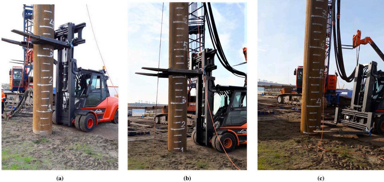
Fig. 9. (a) First, (b) second and (c) third installation phases of an ATP.
