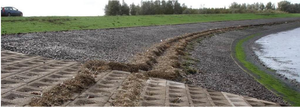
Figure 1. Prototype PBA revetment (Bathpolder, the Netherlands)
