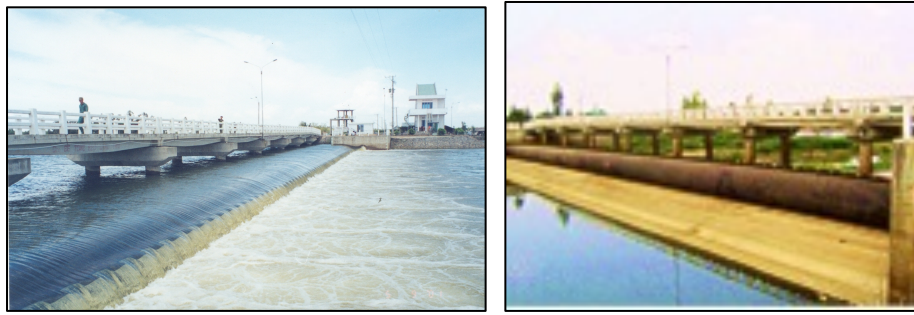
Figure 2-8 Tra Su rubber dam. Right picture shows water flowing over the inundated rubber dam. Left picture shows the rubber dam inflated during the dry periods
