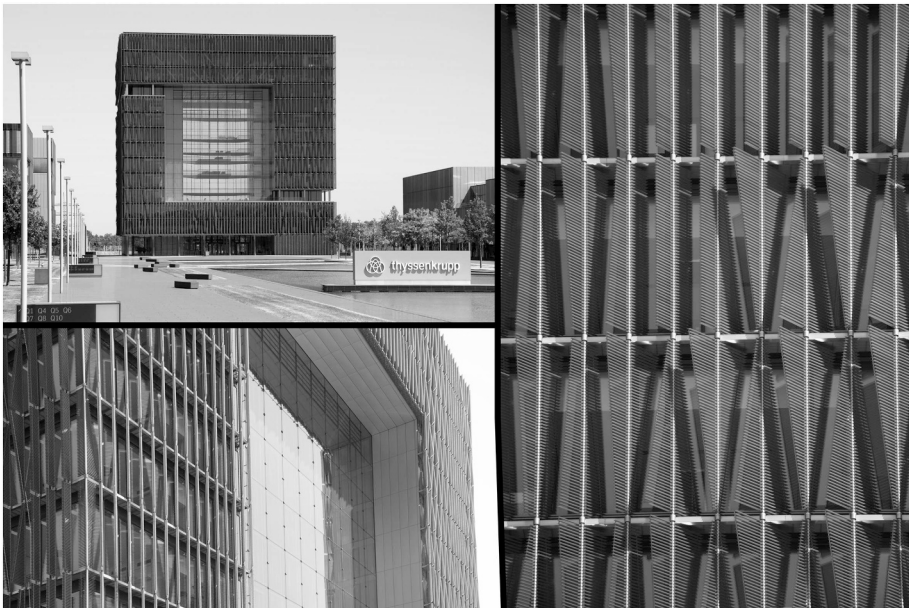
Fig. 5. Q1 Thyssen Krupp Headquarter.
