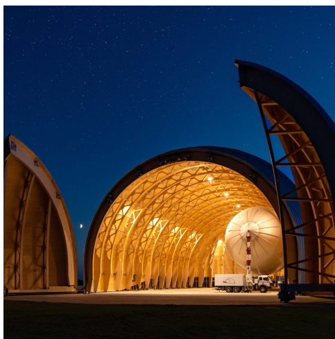
(a) Exterior view of the Luftschiffhalle Mülheim. Adapted from VisitEssen (n.d.). https://www.visitessen.de/essentourismus_convention/location_uebersicht_1/conventionLocation_1511224.en.html
