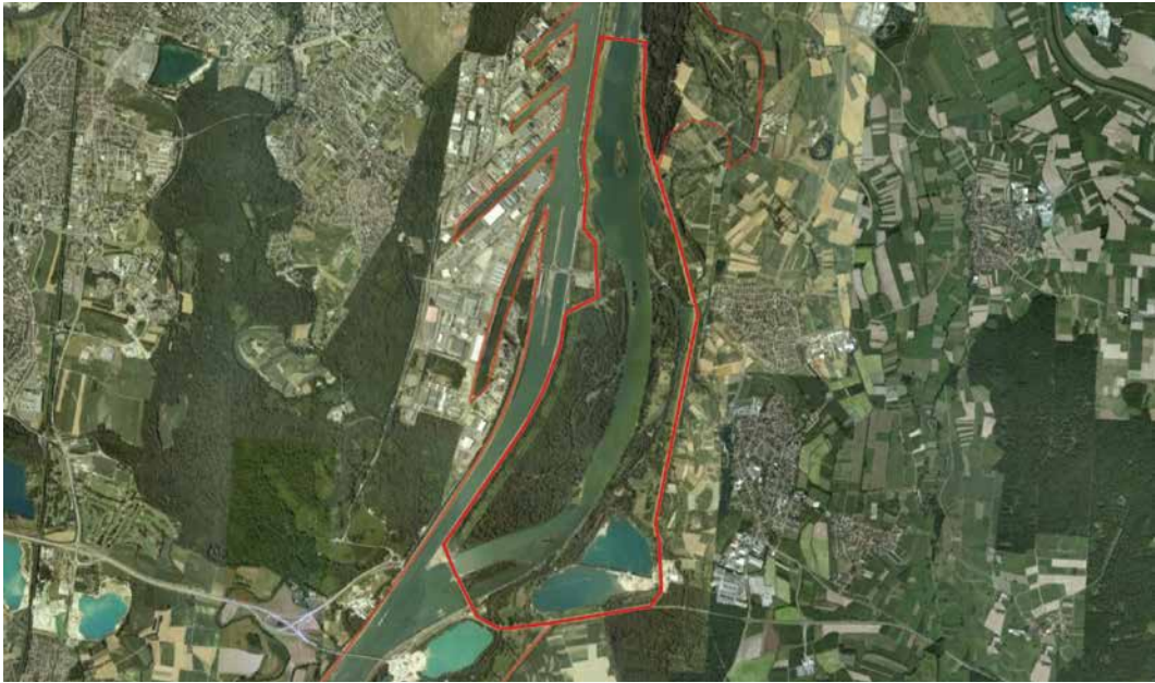
Figure 48 Kulturwehr Kehl/Strasbourg / Rhine km 284-290.2
