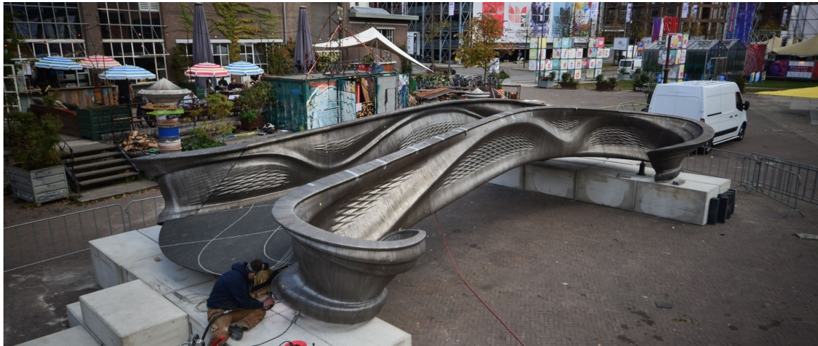
Figure 1.2: MX3D stainless steel printed bridge [3]
