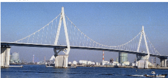
Figure 2 Konohana Bridge Japan
