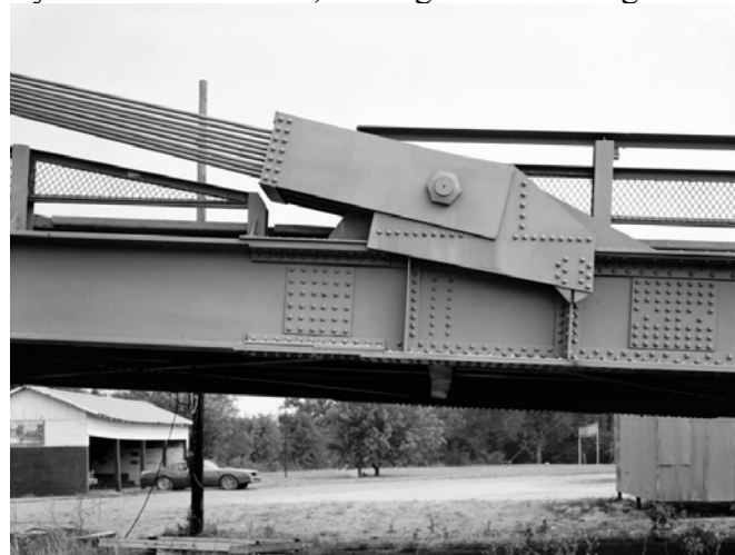
Figure 68 Deck anchorage Hutsonville bridge
