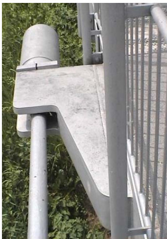
Figure 67 Anchorage of a German footbridge
