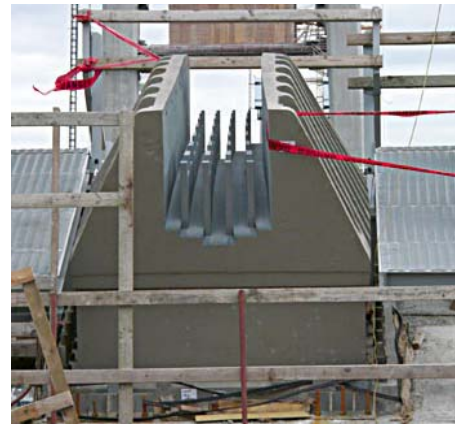
Figure 62 Splay saddle
