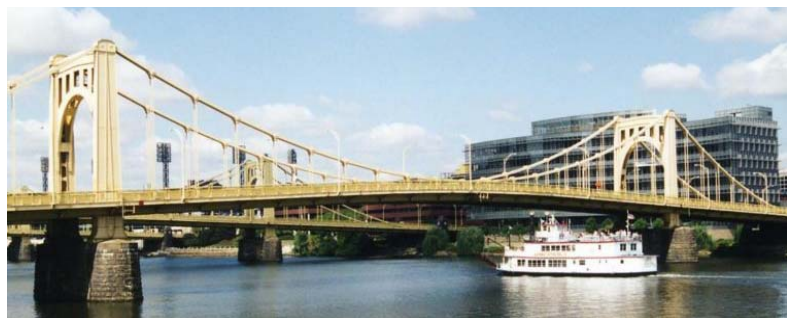
Figure 15 Seventh Street Bridge
