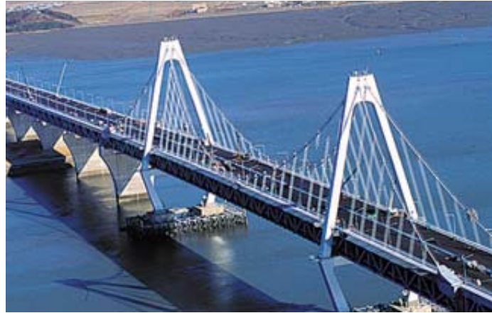
Figure 26 Yeongjong Grand Bridge
