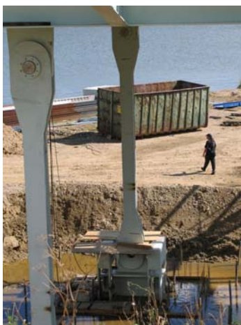
Figure 72 Vertical deck anchorage Kanne Bridge
