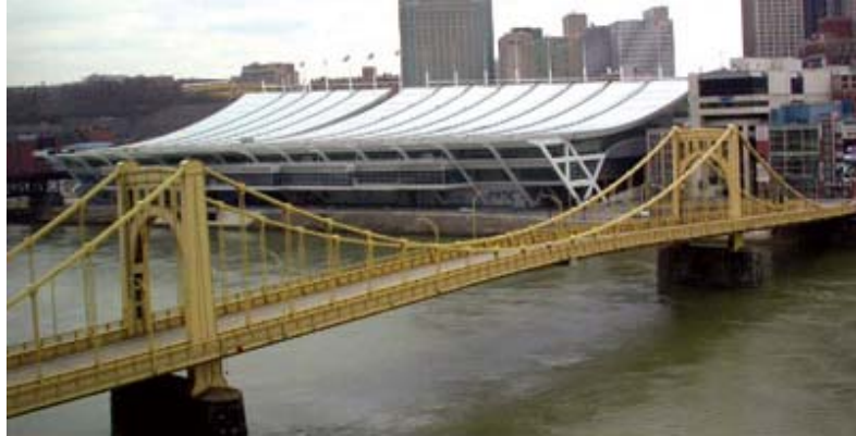
Figure 16 Ninth Street Bridge
