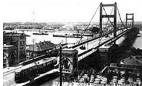
Figure 21 King Alexander 1 Bridge
