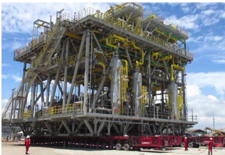
Figure E.6: An example of how the modules will be transported to the right location on site. Obtained by Tata Steel, 2025a.
