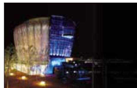
Figure 0.6 Cyclebowl façade. Image courtesy Atelier Brückner.
