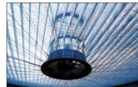
Figure 0.7 Cyclebowl roof system with integrated active daylight system. Image courtesy Atelier Brückner.
