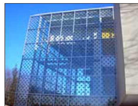
Figure 3.15 Photovoltaic cells in insulating glass panel. Image courtesy Syracuse glass.
