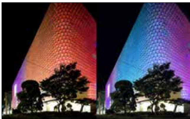
Figure 0.13 Galleria Department store, Seoul, UNstudio, 2003. Image courtesy UNStudio
