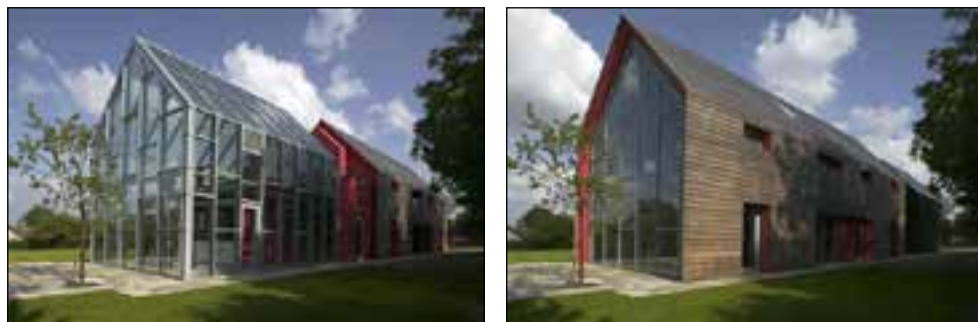
Figure 0.18 Sliding house. Image courtesy dRMM.
