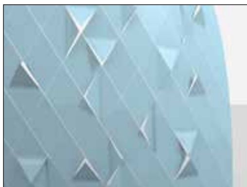
Figure 4.4 Variation of façade tessellation for ventilation and sun accession
