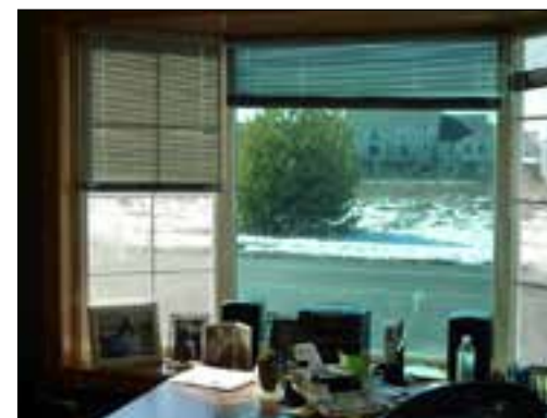
Figure 3.12 Activated thermo-chromic daylight system, with low visual capabilities. Image courtesy by Pleotint.
