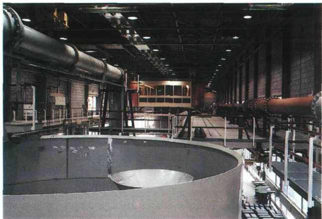
Figure 6 Test sections hydraulic machinery laboratory
