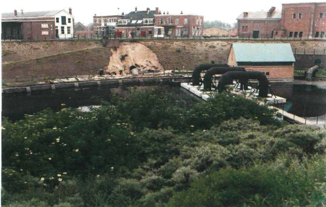
Figure 1 Drinking water pipeline fracture. General view.
