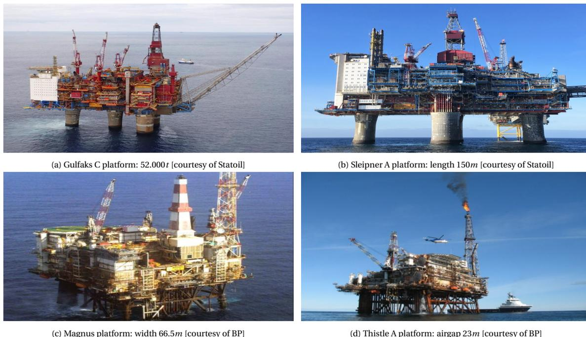
Figure 2.10: Four of the most extreme North Sea platforms
