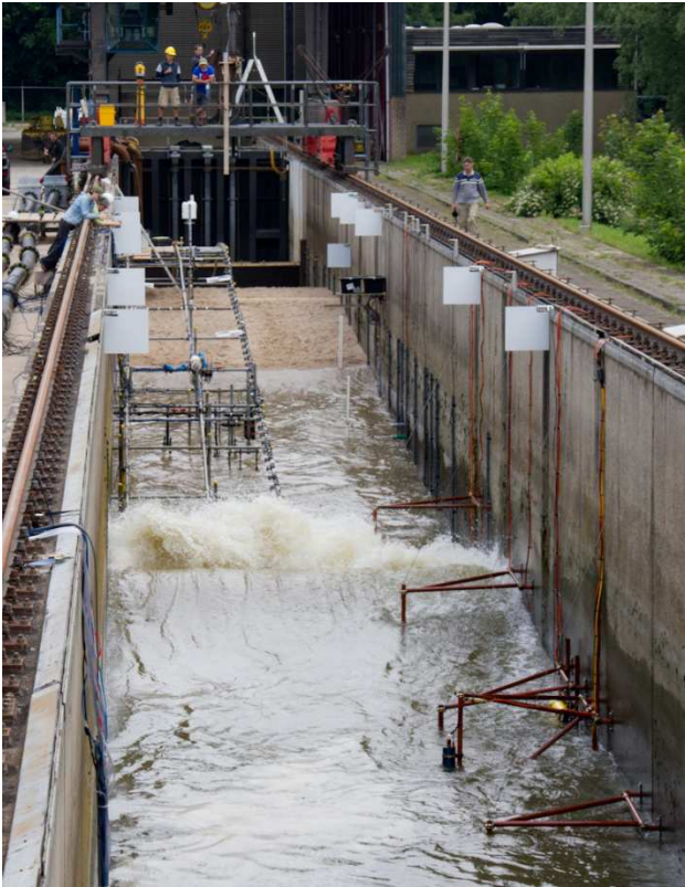
Figure B.4 The barrier during the waves, seen from the 'seaside'
