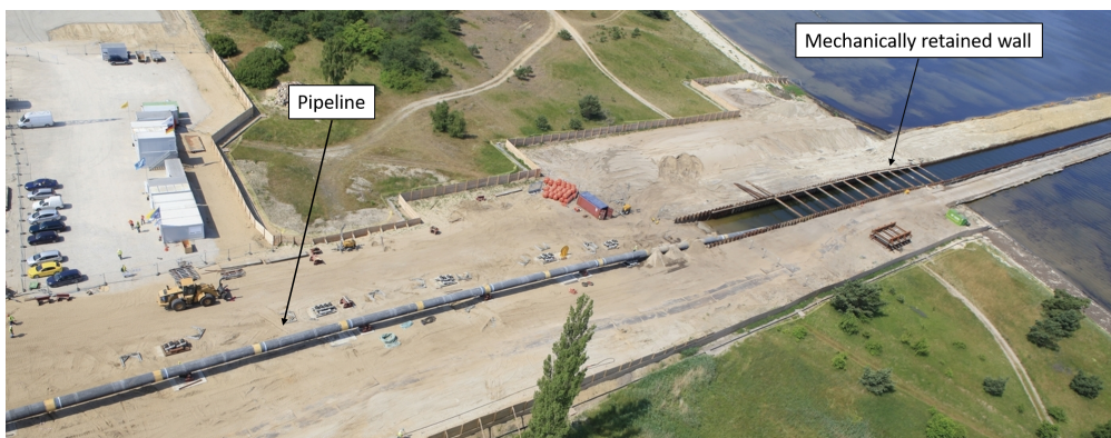
Figure 1.1: Landfall operation through a mechanically retained trench, July 2010, Germany (Nord Stream AG)
