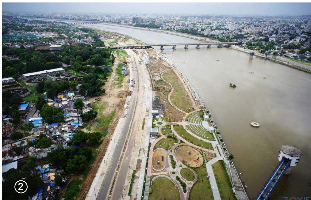
Fig 5.14: Ahmedabad city positives and negatives 1. Water flooding due to excessive rain Source: 5. Public friendly riverfront Source:
