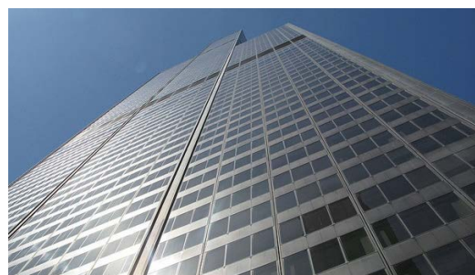
Fig 8.34: Vertical Solar Panels- Chicago Source: http://inhabitat.com/chicagos-willis-tower-to-become-a-vertical-solar-farm/
