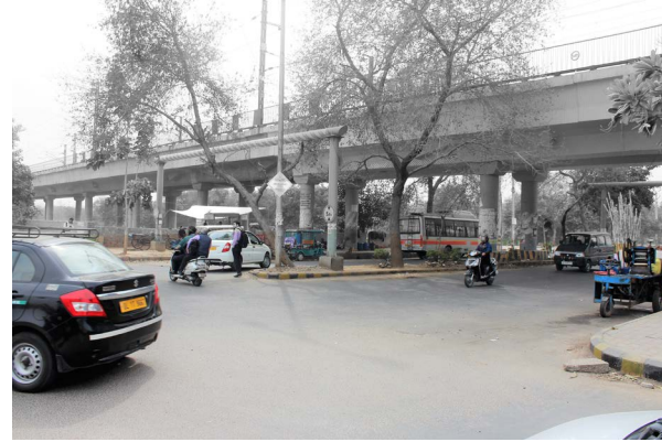
No pedestrian movement pattern on the wider roads. Not safe while walking/ crossing the roads.
