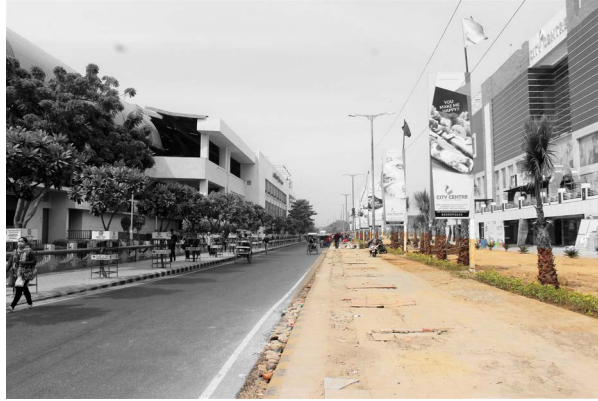
The extra waste space between the road and the buildings. Can be used in a better manner.
