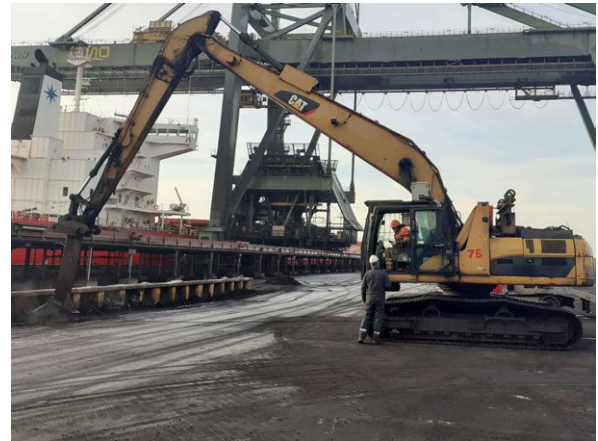
(b) Excavator using the jet attachment to clean a sheet pile wall section
