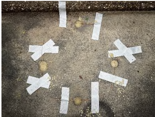
(b) Fresh high-strength mortar after hole filling.
