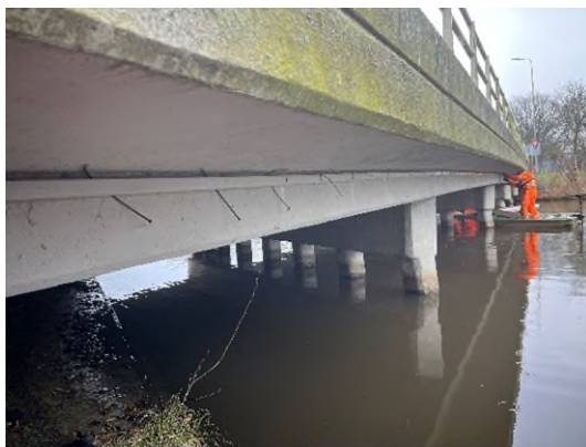
(c) Installation of data acquisition systems and Organizing cables.
