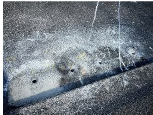
(a) Designated drilling locations after hole drilling.
