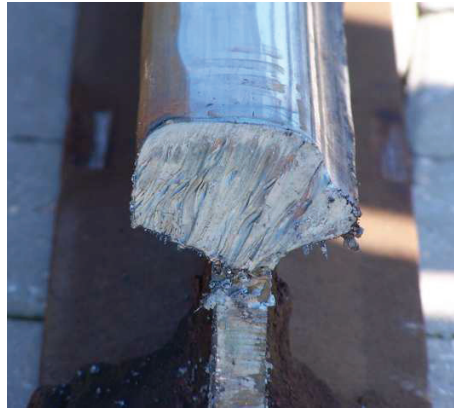
Figure. 6.7: severe wear and downwards plastic flow at the rail gauge corner
