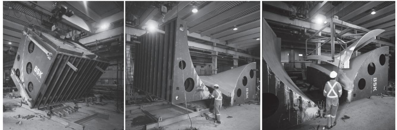
Figure 1.17 Casting process of the half shell elements. [38]
