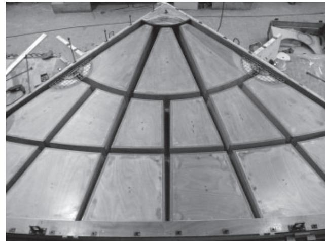
Figure 1.20 Formwork for the elements of the canopy. [64]
