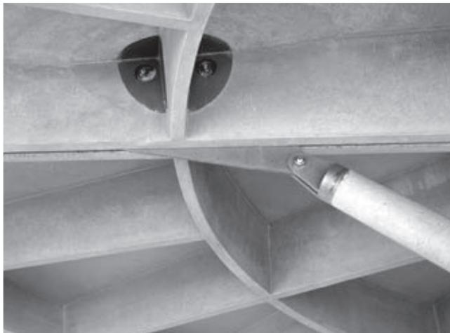
Figure 1.19 Detail of the connection between the branches and the roof. [50]
