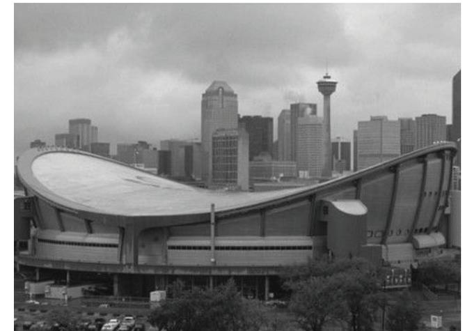
Figure 2.4 The Saddledome (Calgary, 1983) is an example of an anticlastic curved structure. [64]
