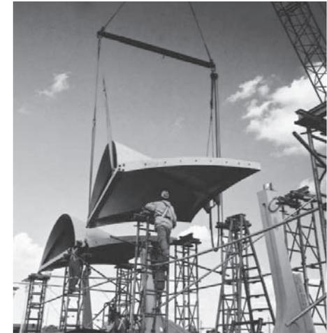
Figure 1.16 Placing of the canopies on the columns. [38]
