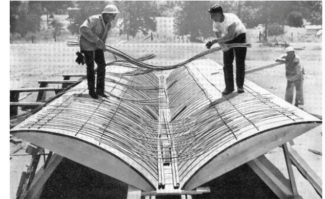
Figure 4.1 Curved reinforcement for a prefabricated concrete element. [20]
