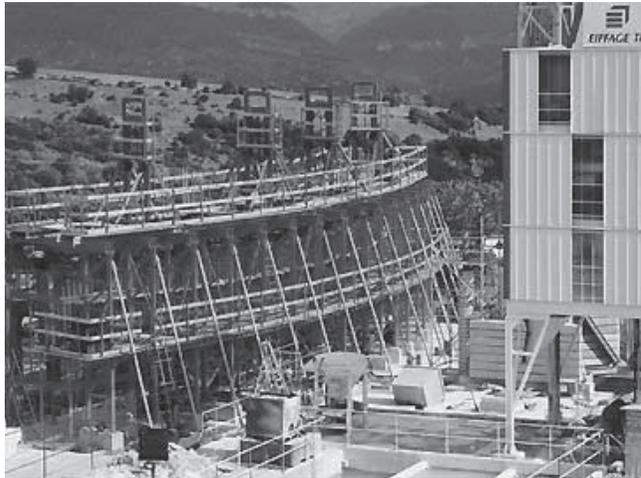
Figure 1.23 On-site casting factory and concrete mixing plant. [61]
