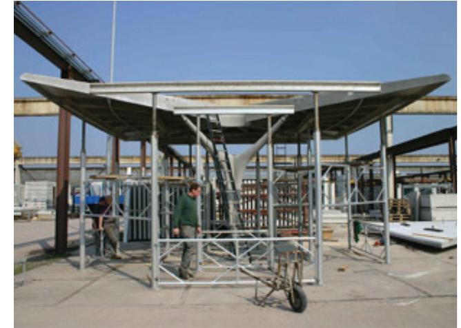
Figure 7.10 Temporary scaffolding used during the construction of the canopy at sanatorium 'Zonnestraal'.
