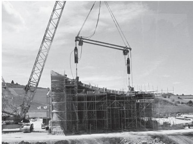
Figure 1.24 Temporary scaffolding for the installation of the precast elements. [64]
