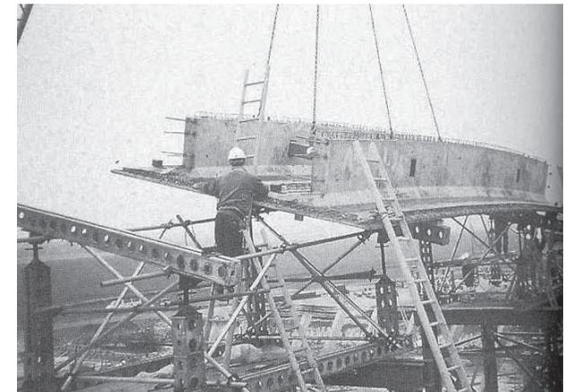
Figure 1.12 Placement of the elements on the temporary scaffolding [28]
