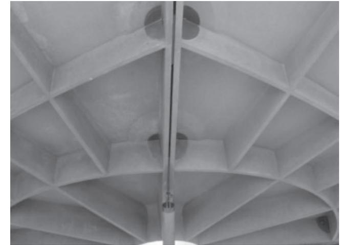
Figure 10.17 Detail of the ribbed elements used for the canopy at sanatorium Zonnestraal.
