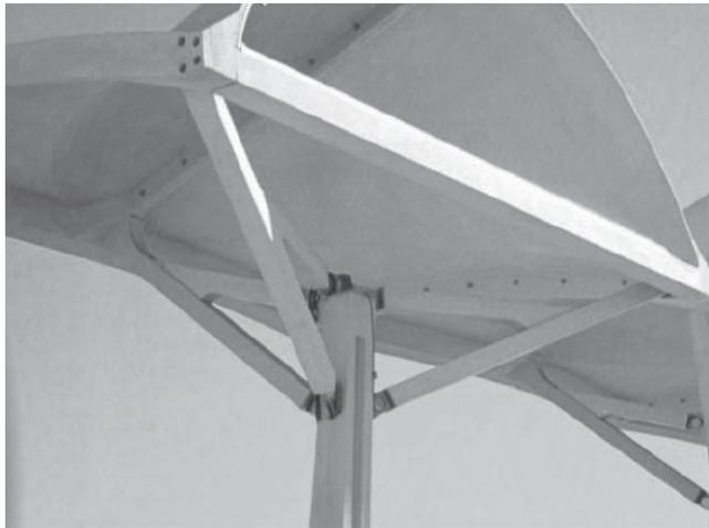
Figure 1.13 The connection between the column and the shell through three struts. [58]
