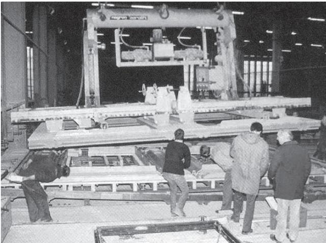
Figure 7.5 A flat element lifted by a vacuum lifting machine. [2]
