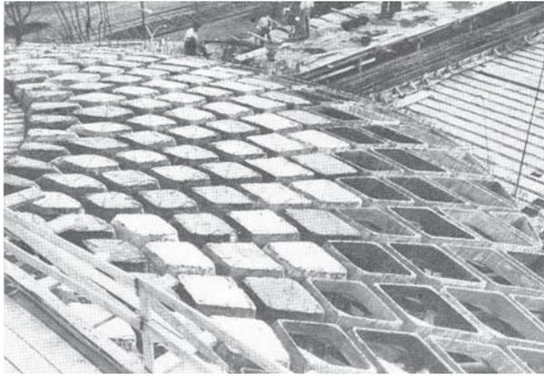
Figure 1.5 Prefabricated pans of the Turin Exposition hall in place, Nervi. [19]
