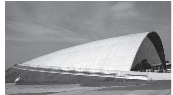
The aircraft museum in Duxford is one of the few prefabricated concrete shell structures.
