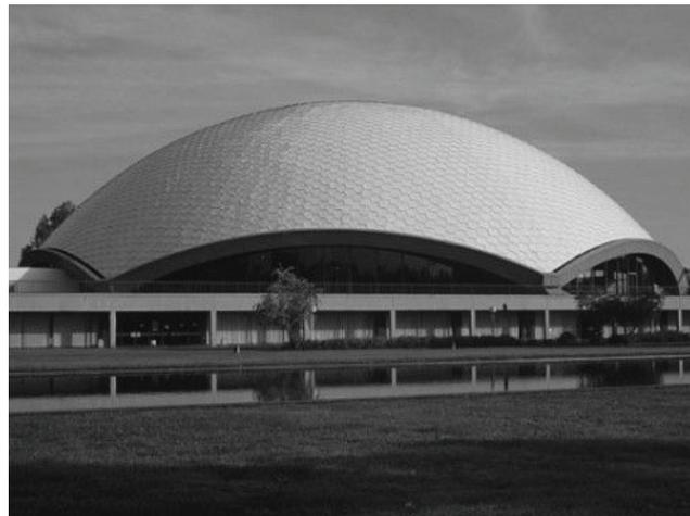
Figure 2.3. The Jahrhunderthalle Hoechst (Frankfurt, 1963) is an example of a sinclastic curved structure. [64]
