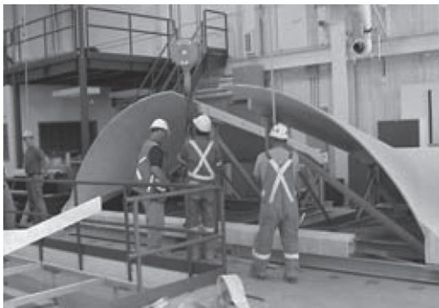
Figure 1.14 The different parts of a canopy before connection. [26]
