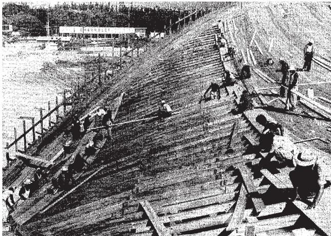
Figure 1.2 Construction of the formwork for a concrete shell structure.
