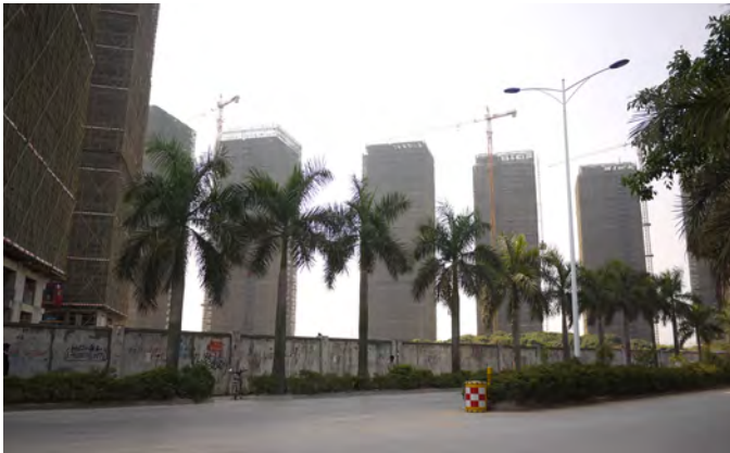
Figure 12. Social housing for relocation of villagers.
