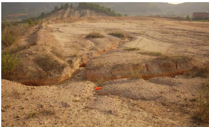
Figure 24. The dike for Gongming Reservoir under construction.
