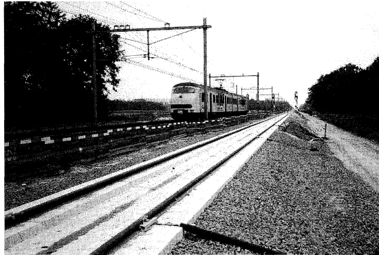
Fig. 3. Embedded Rail Structure installation near Best (the Netherlands)
