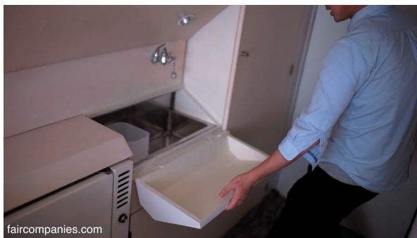
Figure 4-22. The fold-able cooking table in the capsule unit (Dirksen, 2015)
