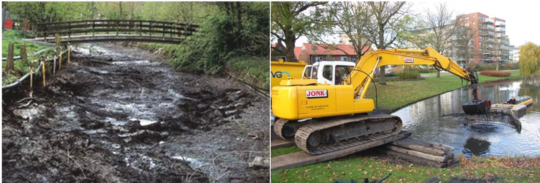
Figure 3.3 Surplus sediment removal.
