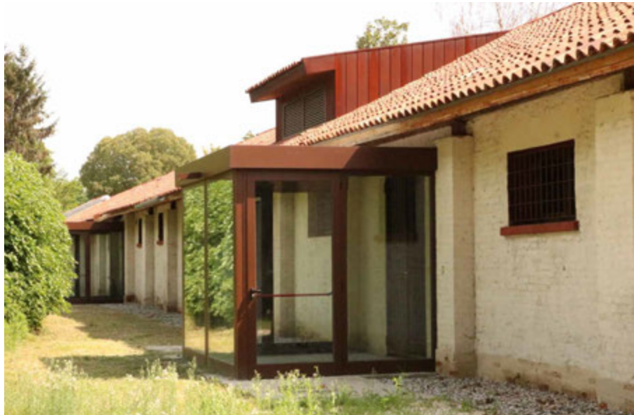
FIG. 5.47 Venice (IT), Forte Marghera: project for the Centro Studi per la valorizzazione delle architetture militari e dei sistemi difensivi (Study Centre for the enhancement of military architecture and defensive systems) (Design: INSULA S.p.A.), building 53: northern façade after the intervention (2015-2017) (F.Marulo 2020)
