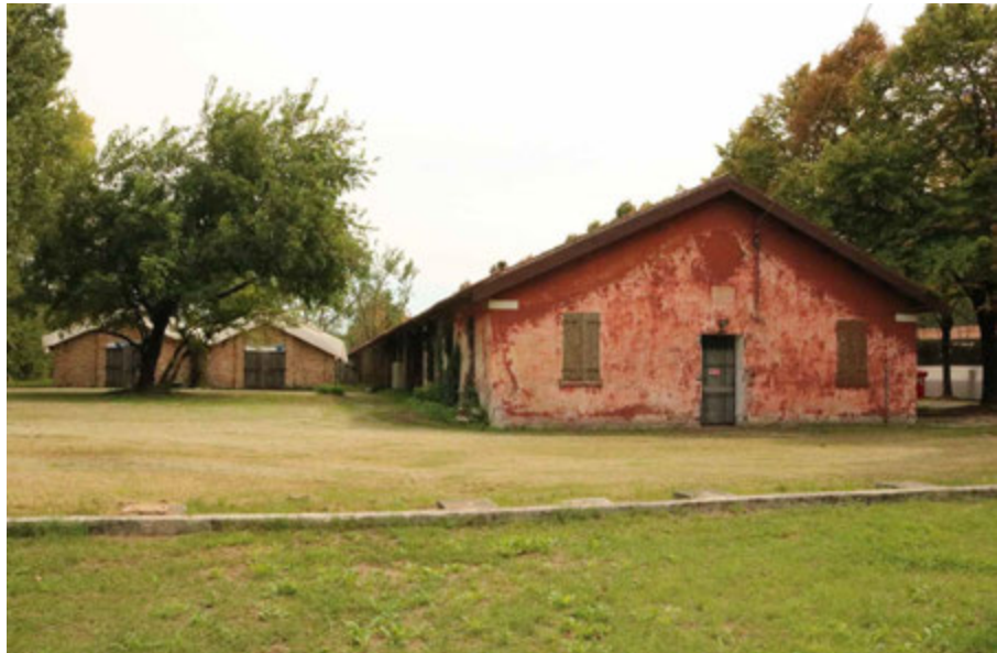
FIG. 5.48 Venice (IT), Forte Marghera, buildings 35-36: northern façade (F.Marulo, 2020)
