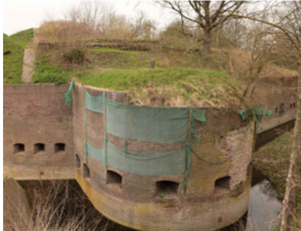
FIG. 4.42 Bunnik (NL), Fort bij Vechten. Central redoubt: exterior (back) after the intervention (F. Marulo 2019)
