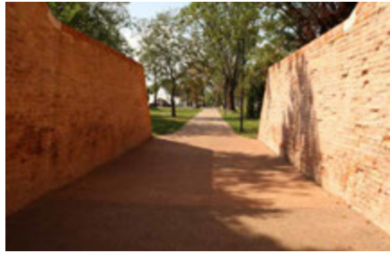
FIG. 5.56 Venice (IT), Forte Marghera, central redoubt: recovery of pathways (F. Marulo, 2020)
