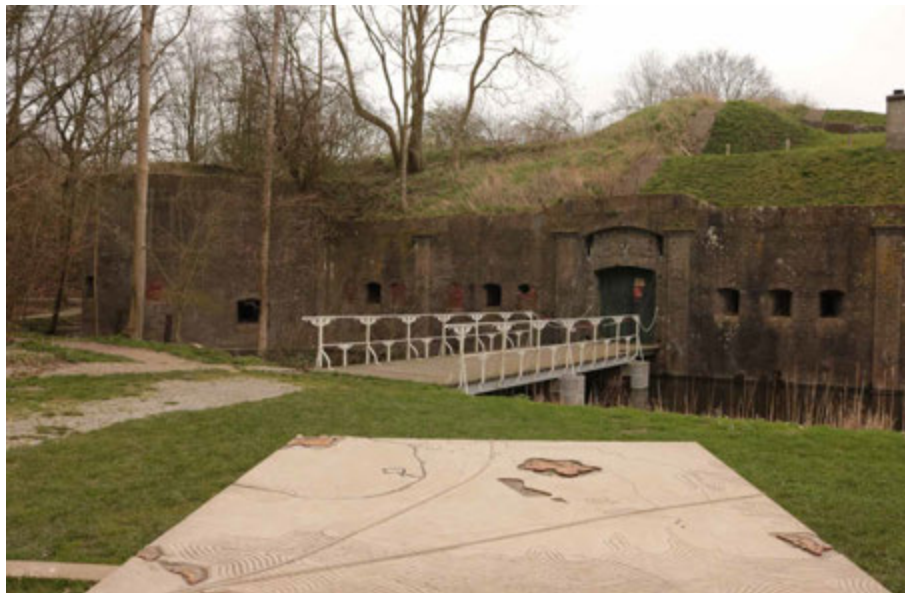
FIG. 4.41 Bunnik (NL), Fort bij Vechten. Central redoubt: exterior (front) after the intervention (F. Marulo 2019)
