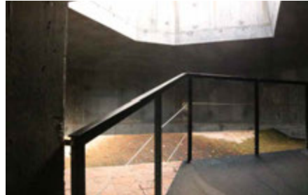
FIG. 4.53 Bunnik (NL), Fort bij Vechten. Flank battery EL: the opening on the roof seen from the outside (F. Marulo 2020)
