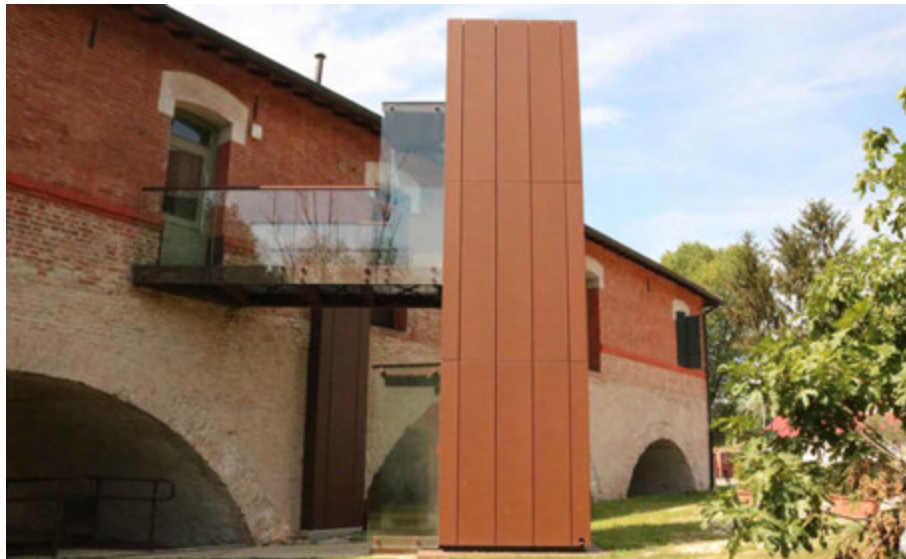
FIG. 5.44 Venice (IT), Forte Marghera: project for the Centro Studi per la valorizzazione delle architetture militari e dei sistemi difensivi (Study Centre for the enhancement of military architecture and defensive systems) (Design: INSULA S.p.A.), building 1: view on the rear façade with the new external elevator after the intervention (2015-2017) (F.Marulo 2020)
