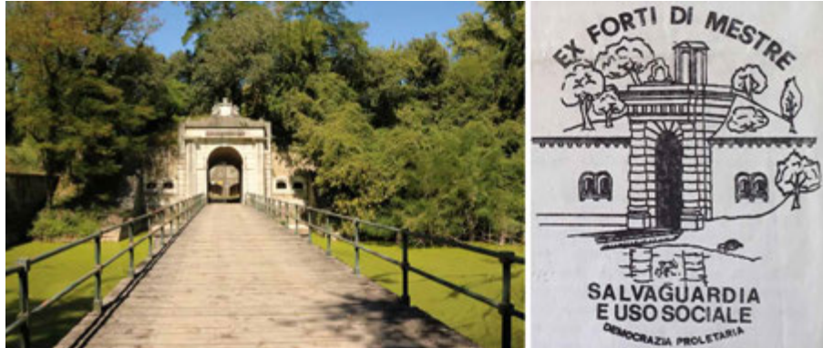
FIG. 5.18 Venice (IT), Forte Gazzera: the monumental portal characterizing the three forts of first generation (left, F. Marulo 2020), used by the local associations as a symbol of the revitalization of the Entrenched Field of Mestre (right, 1984) (ACCTM, Fond 1, Box Coordinamento per il Recupero del Campo Trincerato di Mestre , File 2)
