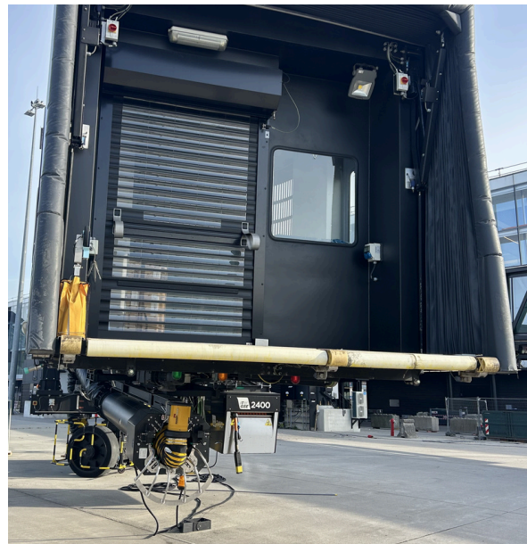
Figure 2.6: Electric ground power configurations at Schiphol: standing FPU on island (left), an FPU mounted underneath the PBB at the A-pier (centre), and a mobile e-GPU (right)
