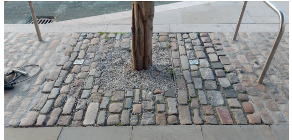
Fig 31, Tree pit design, granary square London (2023)
