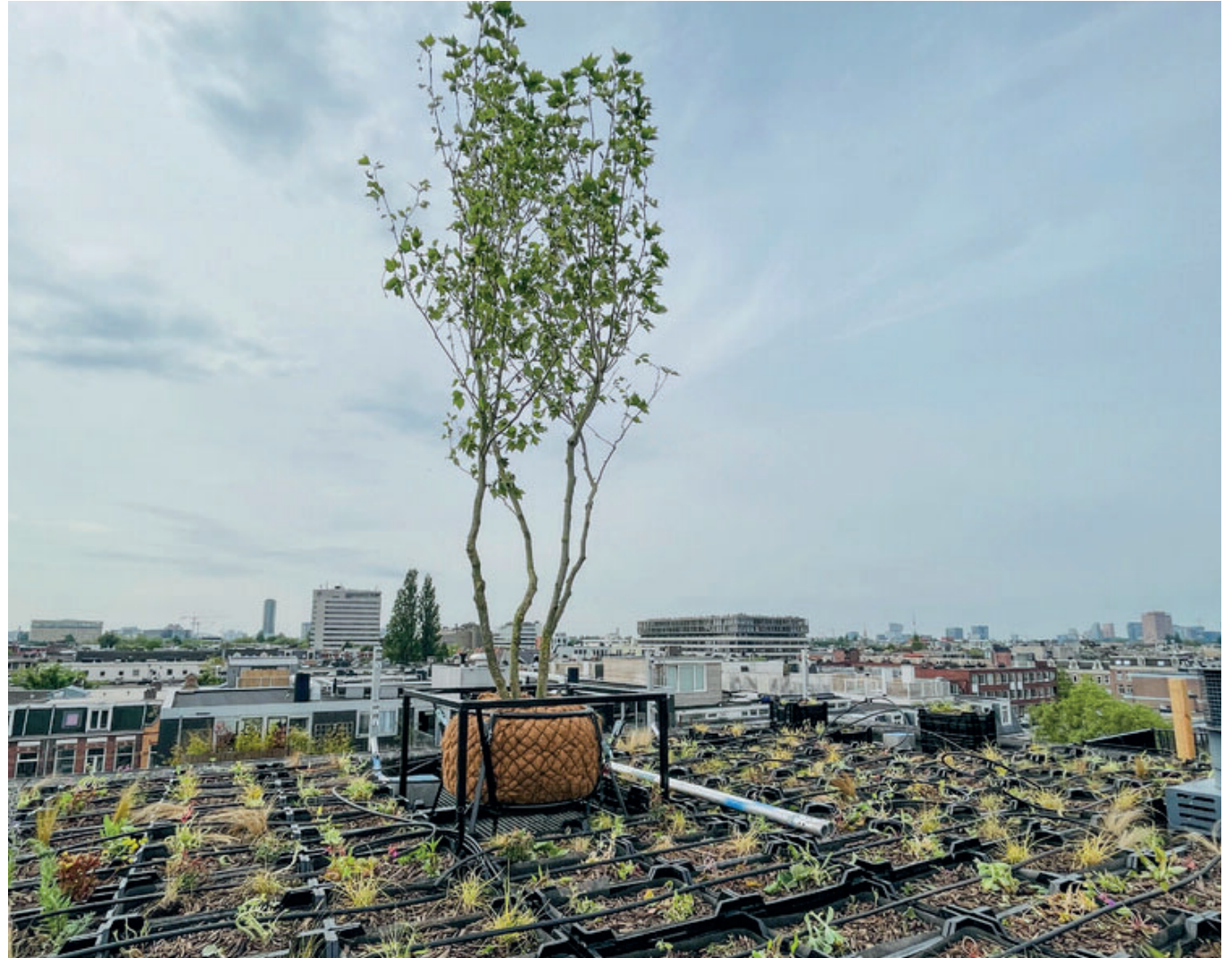
Fig 36, Rooftop tree design by Urban Jungle project (2023)
