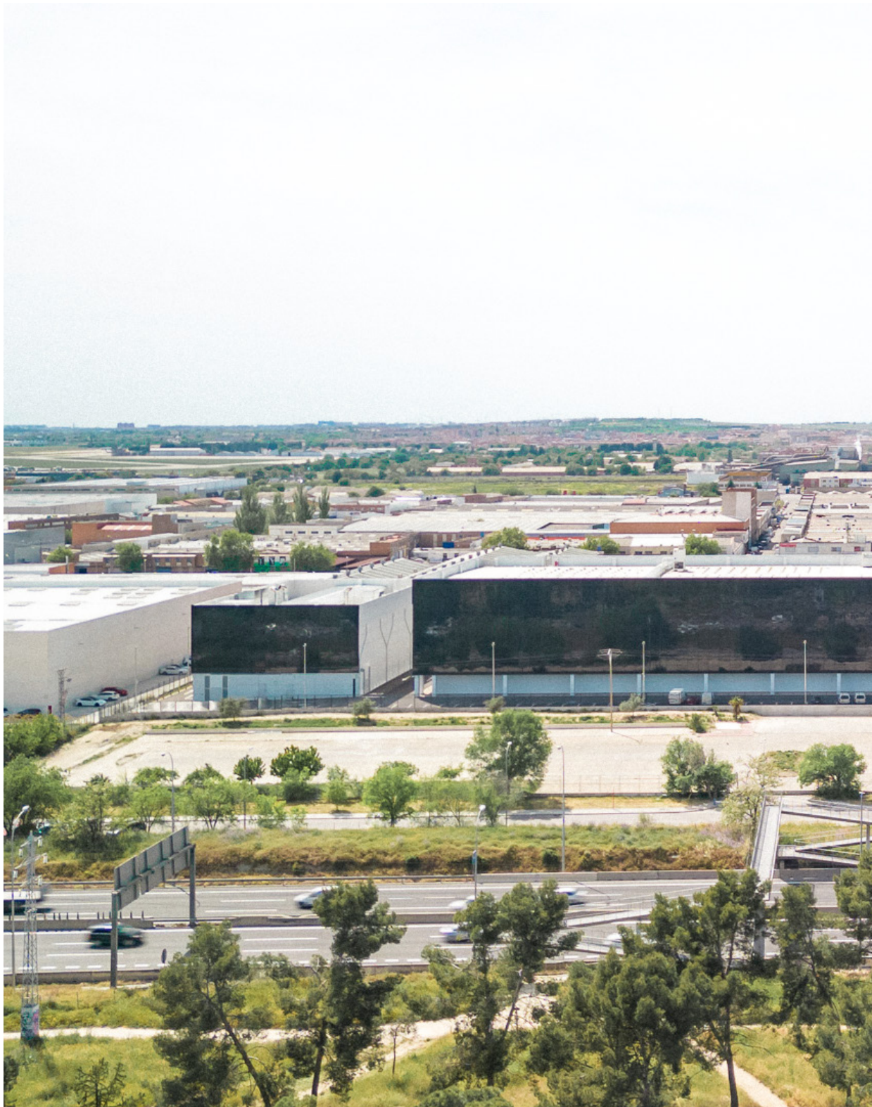
Figure 2 / Merlin Data Center / Getafe / Madrid / Spain / MerlinProperties, 2015
