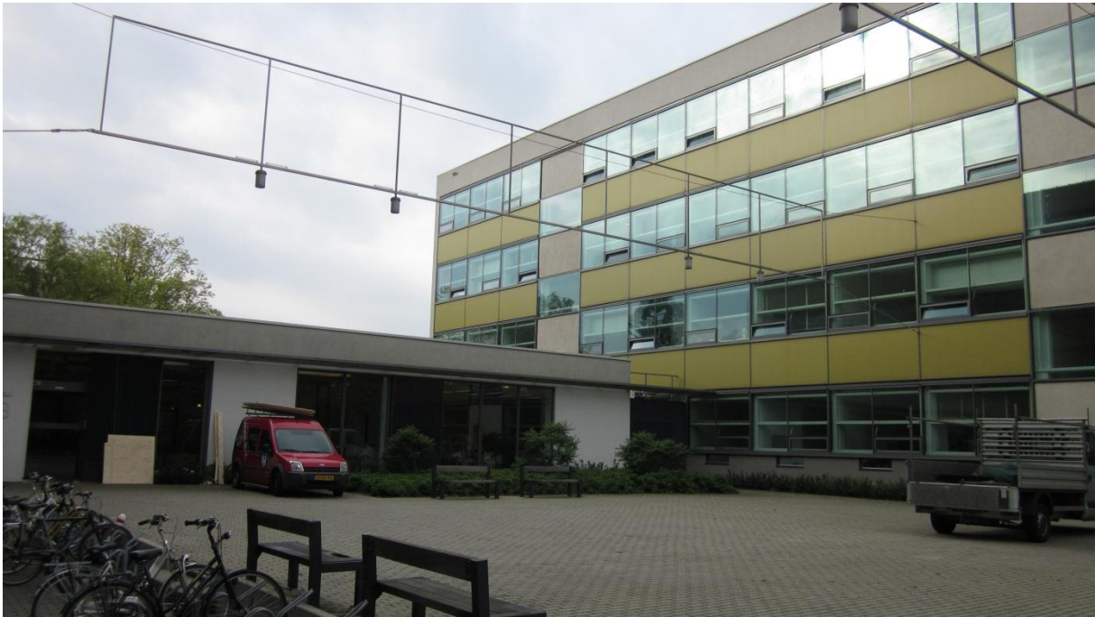
Figure 20. Photo of wing 2 and wing 3 of the OTB building
