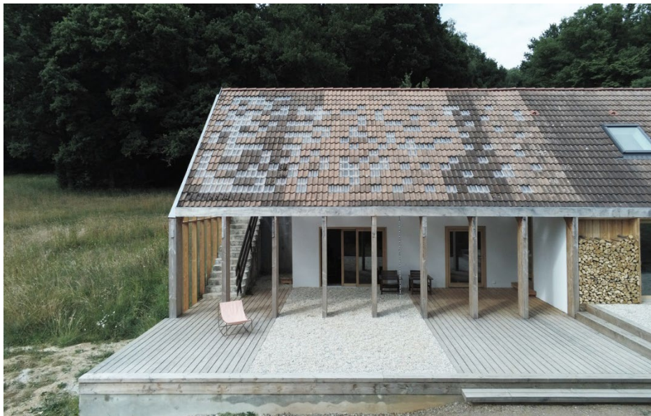
Figure 6. Once Upon a Time in the Perche House by Java Architecture. (Dethier, no date).
