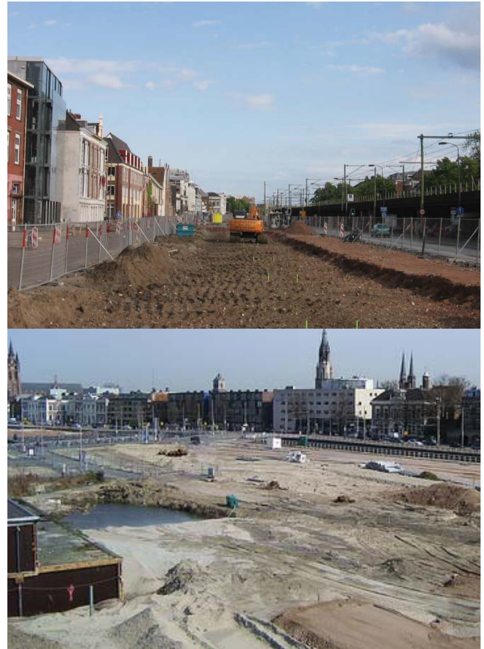
fig 9.29: Building process in Delft
