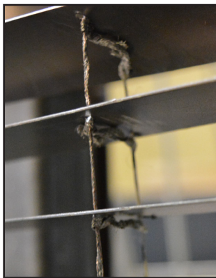
Photo 4: keeping the lamellae in place by making a metal ladder cord
