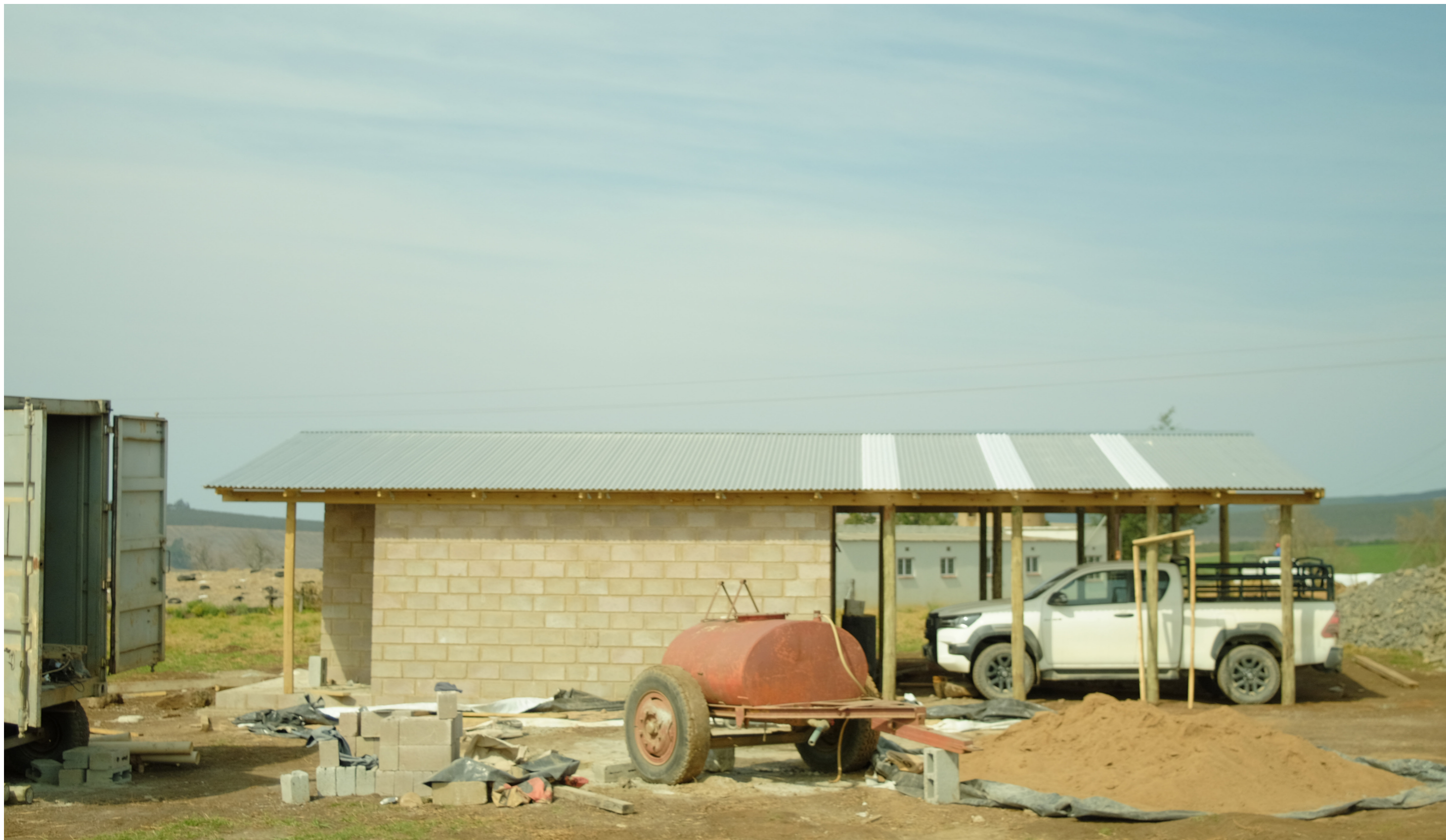
Construction, Rockfontein Farm Anna Hauff, 2025
