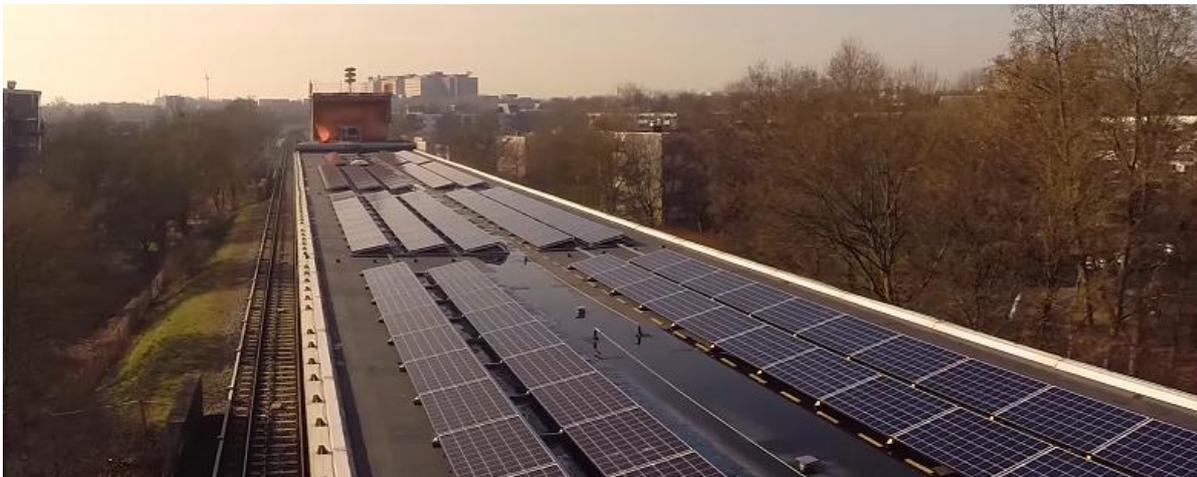
Figure 1.1: 83 kWp PV system on roof of metro station Reigersbos [6]
