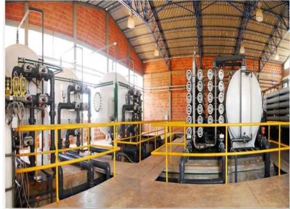
FIGURE 22 DESALINATION PROCESS PRO ACTIVA
