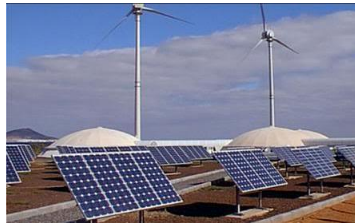
CANARY ISLAND DESALINATION SYSTEM
