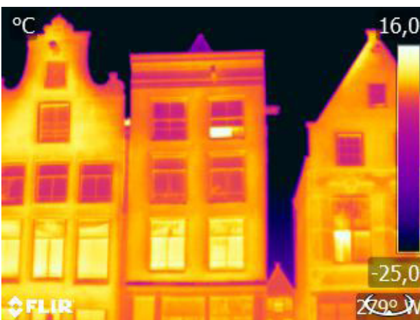
Figure 29: Infrared image of the exterior. Own picture.
