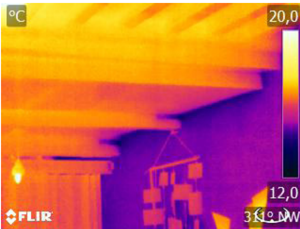
Figure 25: Infrared image of the front house. Own picture.
