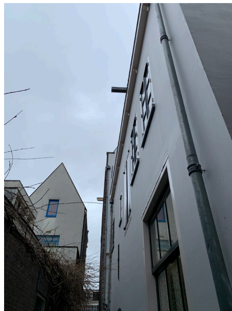
Alley on the North side of building (Suikerbakkersteeg). Own picture.
