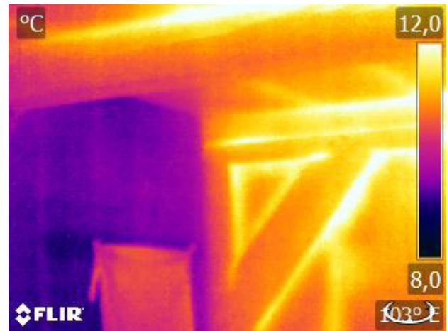
Figure 26: Infrared image of the back house. Own picture.
