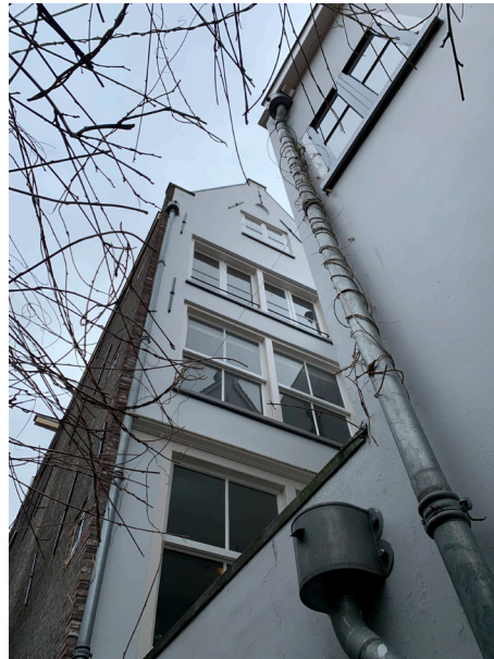
West facade of the front house. Own picture.
