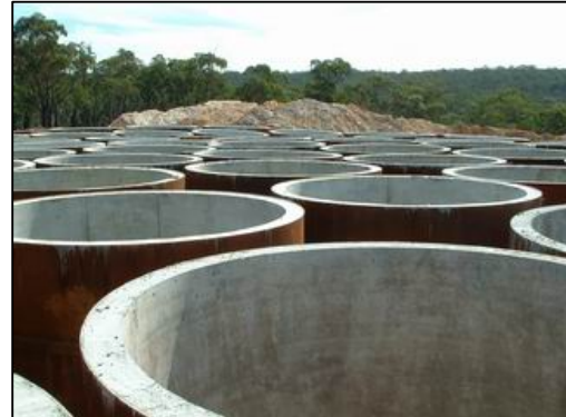
Figure 23 - Composite pre-cast liners ready for floating into a mud-filled shaft.
