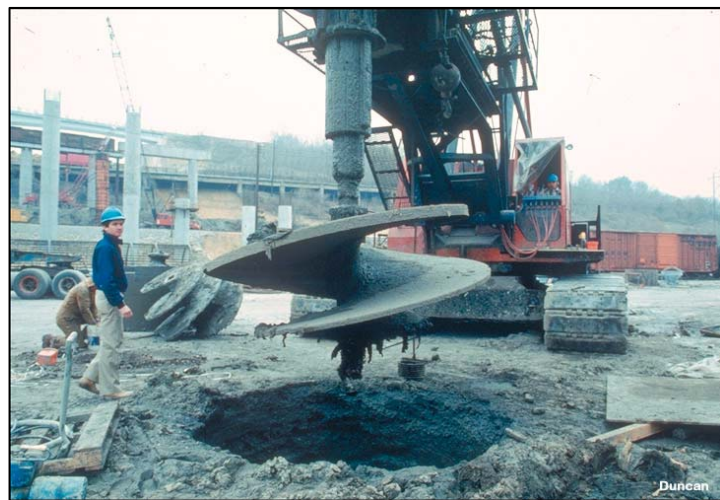
Figure 32 - Excavation of a shaft with a large diameter auger.
