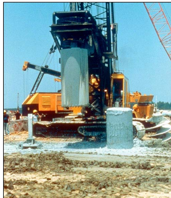
Figure 31 – retrieved segment of core from calyx drill
