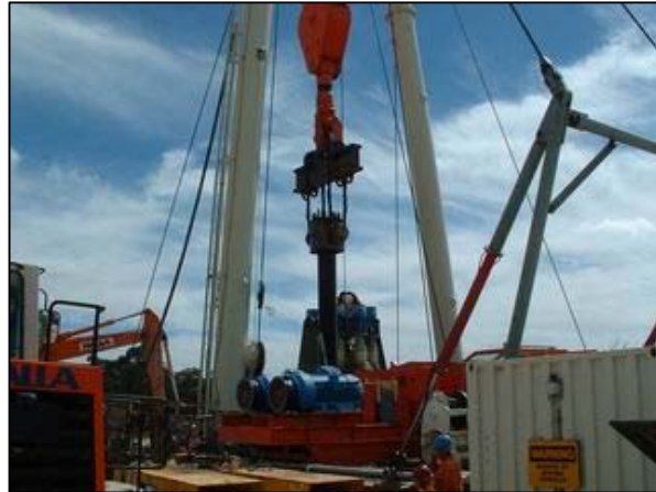
Figure 33 - Headframe for shaft drilling
