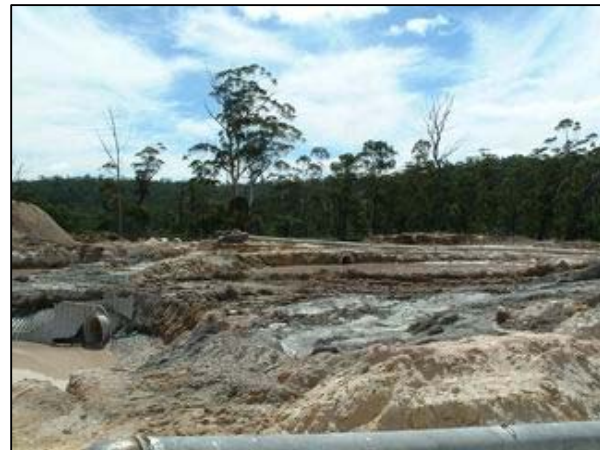
Figure 37 - Settling ponds for drilling mud
