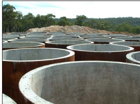
Figure 34 - Composite lining elements which will be welded together as they are floated into the shaft.
