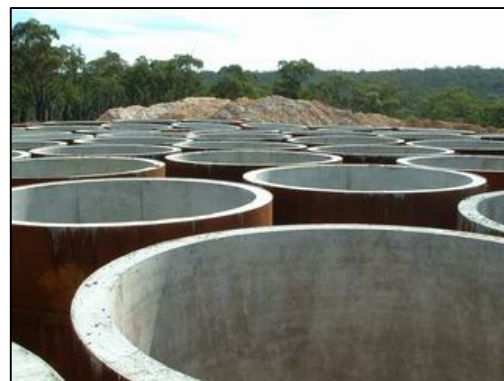
Figure 18 - Composite pre-cast liners ready for floating into a mud-filled shaft.
