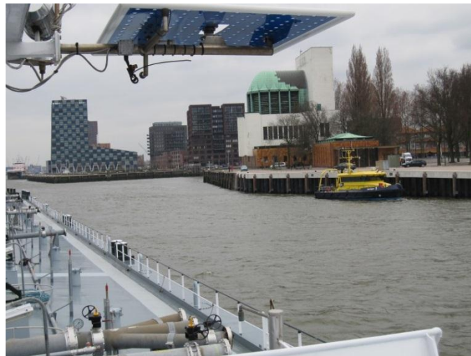
Figure B.4 Survey boat measuring scour depth near quay
