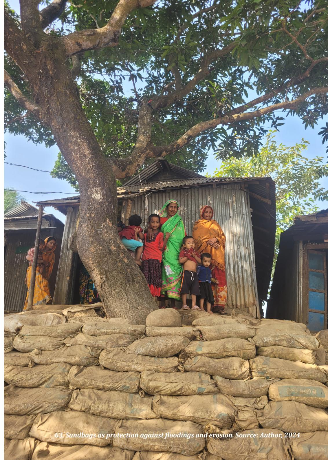
63. Sandbags as protection against floodings and erosion. Source: Author, 2024
