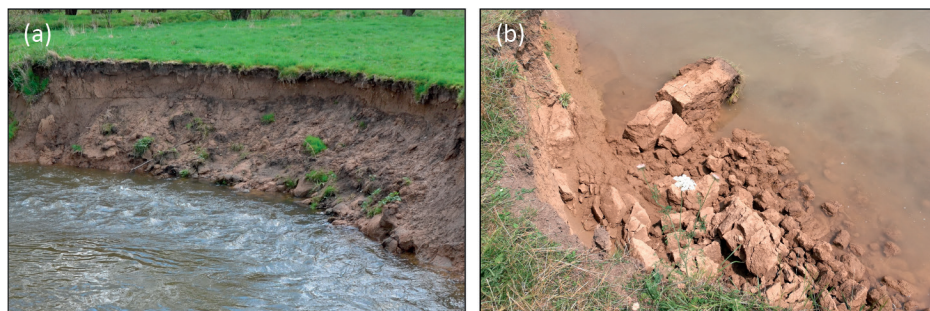
Figure 1.6. Slump blocks at (a) Geul and (b) Meuse Rivers, the Netherlands, respectively resulting from planar and toppling failures.
