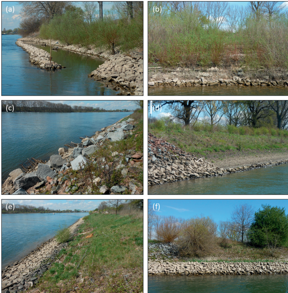
Figure 1.10. Nature-friendly bank protections in test sections on the Rhine River near Worms, on 12/04/2016, after 4.5 years of installation. (a) Stone pre-bank, shallow water zone with dead trunks, and bank with riprap, willow branch cuttings, living fascines, and brush and hedge layers. (b) Willow brush mattresses transversally installed. (c) Riprap with gravel fill, groups of individual stones, and dead wood fascines. (d) Reed gabions and stone mattresses on granular filter, plant mats and hedge layers (note riprap with dead wood on the left). (e) Riprap with top soil alginate mixture, hydroseeding, and individual plants. (f) Riprap and pavement with reeds. Descriptions based on Heibaum and Fleischer (2015).
