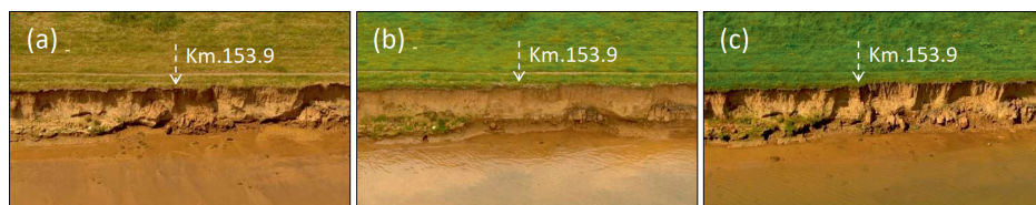
Figure 2.11. Zoomed-in UAV photos from track 1 at section 4, kilometre 153.9, showing diverse bank erosion stages: (a) slump blocks at bank toe on June 21, (b) clean bank face after block removal on July 19, and (c) undermining on August 23.
