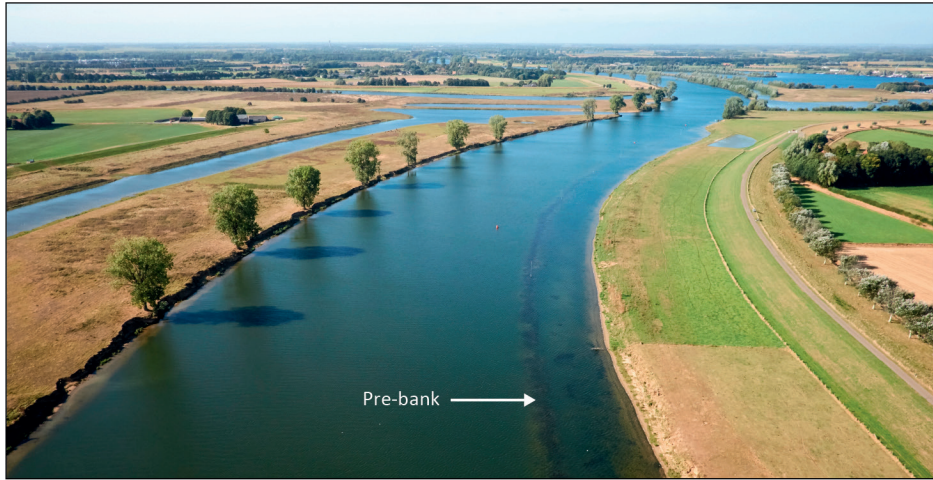
Figure 1.11. Example of a submerged pre-bank protection at Balgoij, the Meuse River, constructed in 2012 to reduce erosion in front of the dike on the right-hand side (28/09/2016). The left eroding upper bank had the riprap removed in 2013 from 0.5 meters beneath the regulated water level. Source: Rijkswaterstaat/J.v.Houdt.
