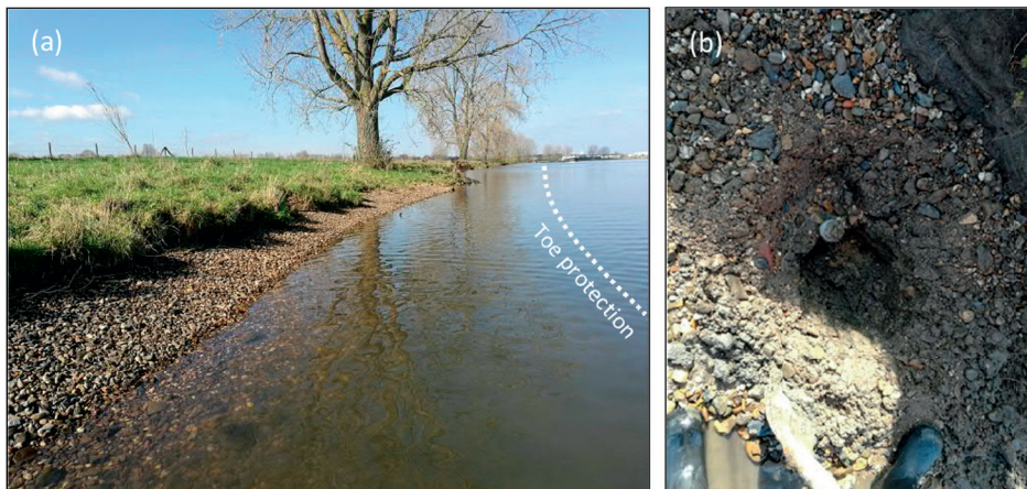
Figure 5.2. (a) Downstream view of re-naturalized bank at Sint Agatha, presenting an armoured terrace. (b) Terrace top soil next to upper-bank toe, composed of a gravel-sand mixture.
