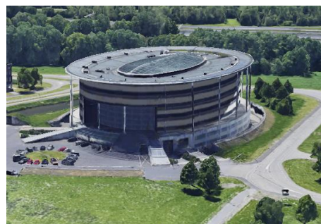
Figure 3.7: Building number 4, HUB 50
