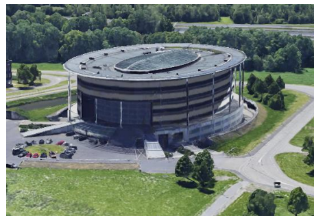
Figure 5.6 Building number 4, HUB 50
