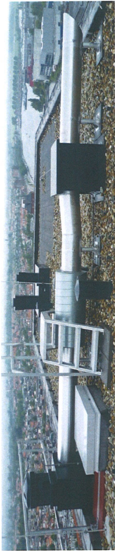
image / figure 2: Ventilation shafts on the roof of the building. In the background the header of a chimney.
