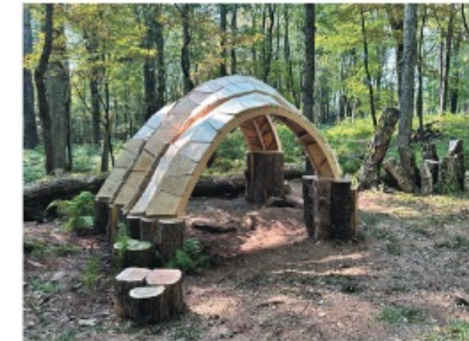
Bio-welding creating thicker panels (24 mm, 48 mm, and 72 mm) with improved stiffness and load distribution
