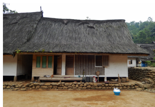
Figure 17: Facade Kampung Naga house (Image by Author)
