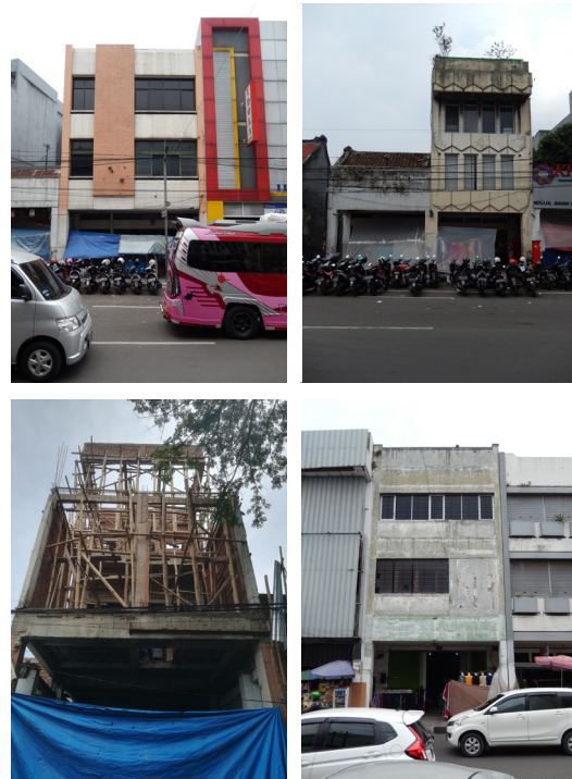
Figure 67: Facades and construction of contemporary shophouses (Images by Author)
