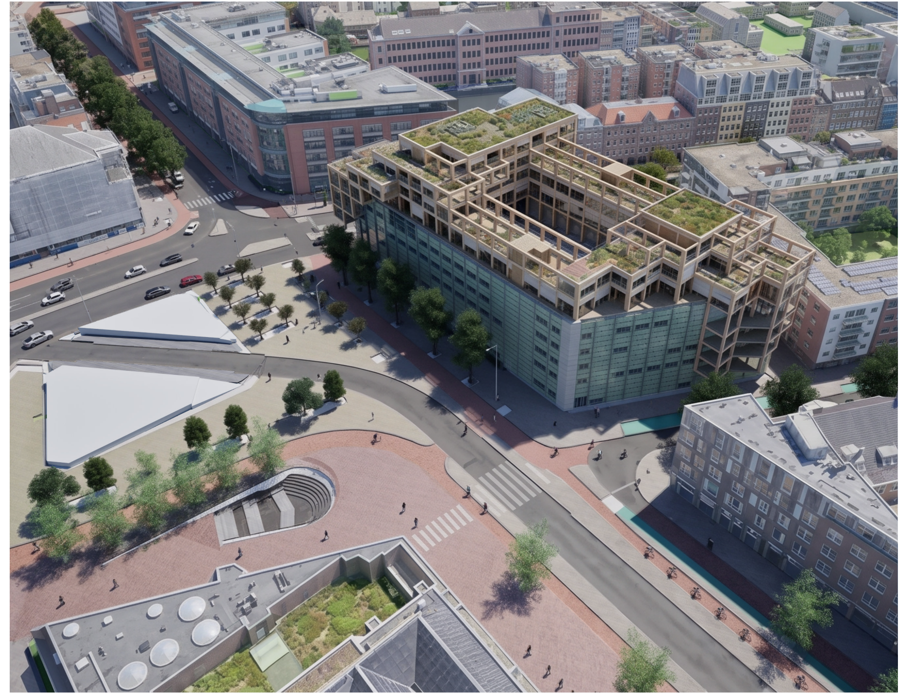
New Extension, View from above
